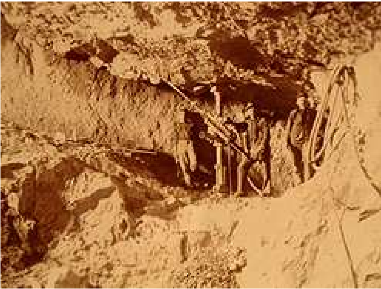
New York & Rosendale Cement Co.: drillers at the Black Smoke Mine. Photo provided by Century House Historical Society, Jeff Kraus Collection
