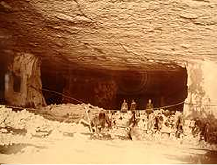
New York & Rosendale Cement Co.: the Black Smoke Mine. Photo provided by Century House Historical Society, Jeff Kraus Collection
