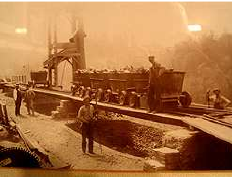
New York & Rosendale Cement Co.: at the top of the kilns. Photo provided by Century House Historical Society, Jeff Kraus Collection
