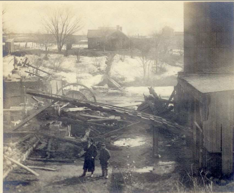
Mill No 1 Fire March 4, 1910 Remains as seen from hill directly west of mill site showing rock crusher, engines, boilers, and part of a kiln (to the right) [CHHS Collection]
