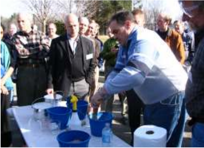
Ken Uraicus mixes up a batch of mortar made with Rosendale Natural Cement
