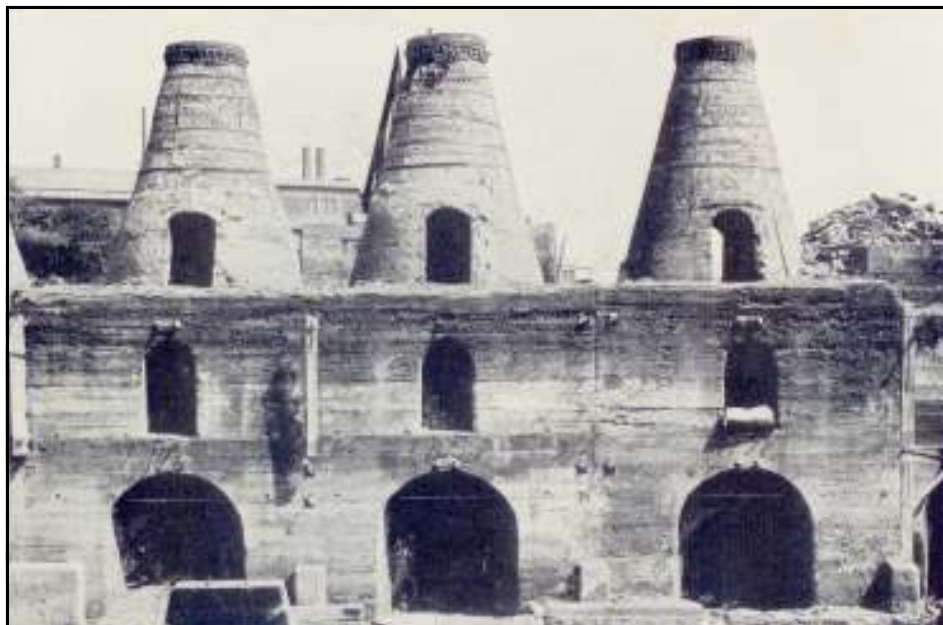
Coplay Cement Company's Schoefer kilns at Coplay, Pa. Erected in 1893. Photo: Radford's Cyclopedia of Construction. 1921.
