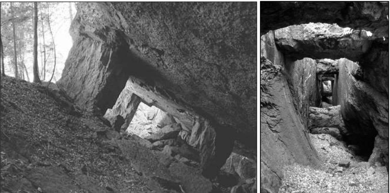
*Examples of steeply dipping (left) and vertical (right) cement mines found in the Rosendale area. The miners followed the folded layers of Rosendale and Whiteport Dolostone. Today these mines provide a unique three-dimensional picture of the local geology.*
