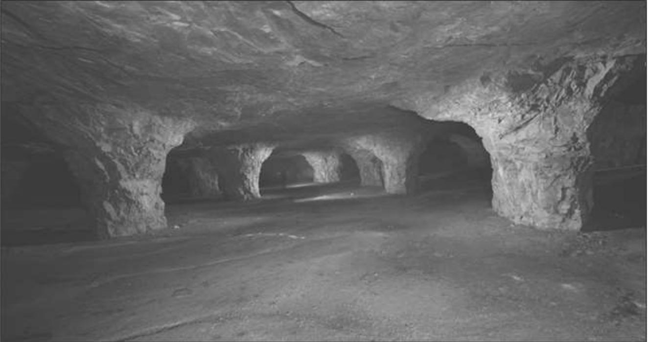
*Relatively horizontal cement mine in the Rosendale area. Columns are composed of the Whiteport Dolostone (which was mined out here) and the roof is a different limestone found above the Rondout Formation (Manlius Limestone Formation).*
